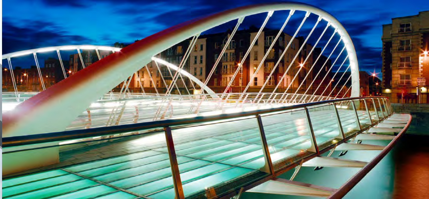
Macalloy Stainless Cable used in Steel Arch James Joyce Bridge; Dublin, Ireland
