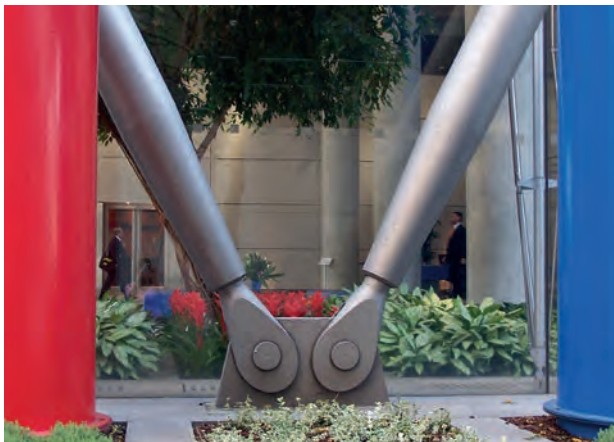
Macalloy's Architectural Adjustable Compression Struts have been used at 88 Wood Street, London, UK
