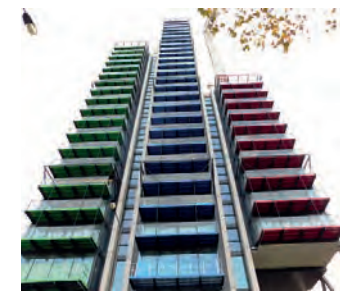
Merano Residences, London, UK. The balconies are being supported by Macalloy Tension Bars
