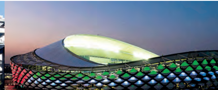
Al Ain Stadium, Al Ain – Macalloy 460 30mm, 42mm & 48mm galvanised bars used as bracing
