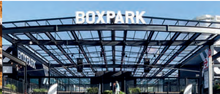
Boxpark – Croydon, UK. M42 Galvanised Tension Rods at 9.9 metres long were used, with central turnbuckles for extra tensioning
